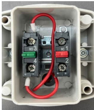
Figure 23: Cabling key switch
